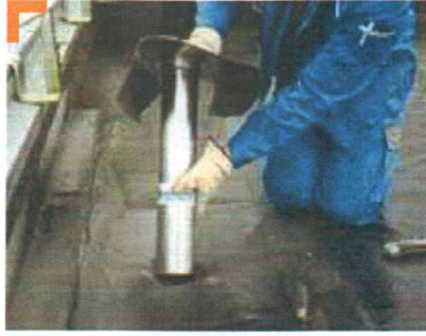
1. Insert Depco into the stack after laying the first layer of waterproofing.
