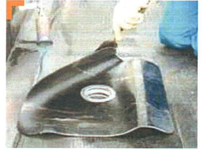
2. Weld the elastomer layer onto the first layer of waterproofing.
