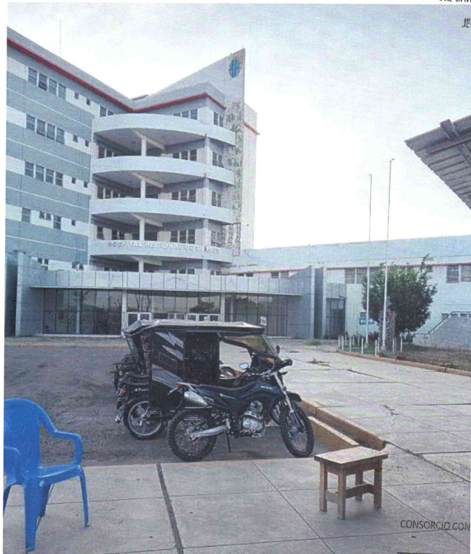
Figura 12-2: Hospital Regional de Tumbes Colapsado
