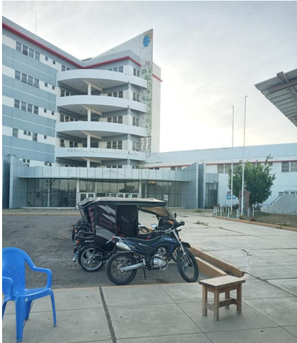
Figura 3-6: Hospital Regional de Tumbes Colapsado
