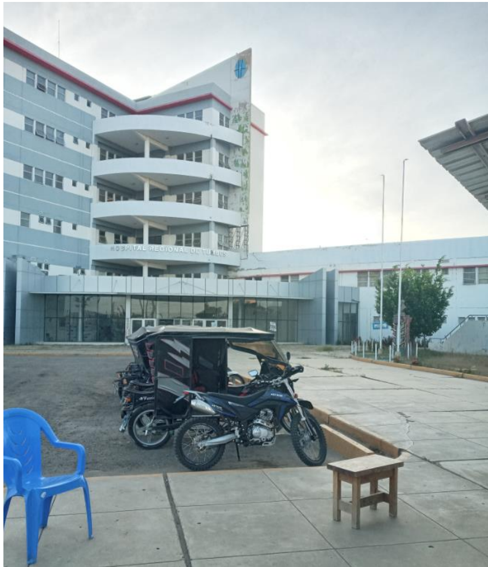
Figura 12-2: Hospital Regional de Tumbes Colapsado
